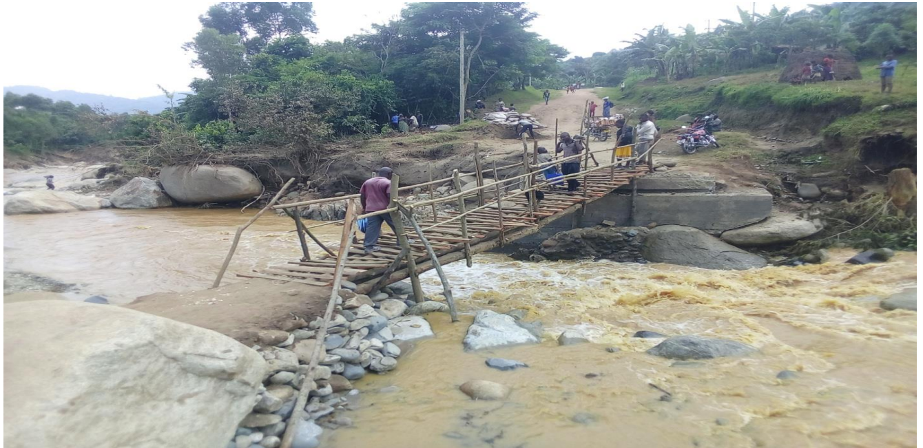
One of the flooded rivers that swept the bridge and community constructed a temporarily one for the mean time
